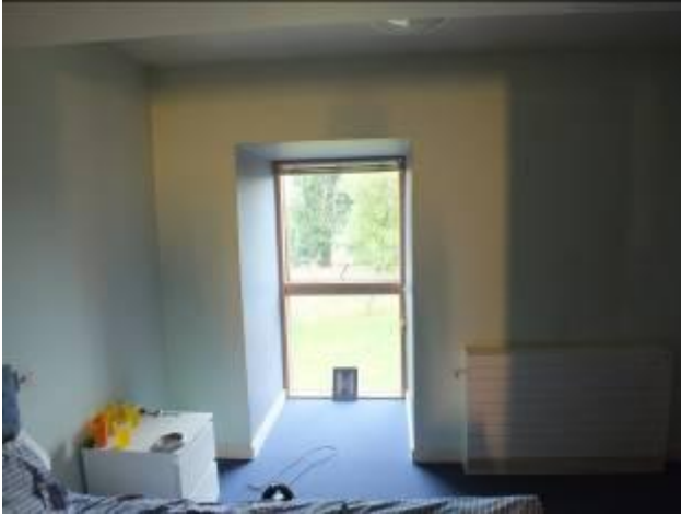
“Pod” window in bedroom
